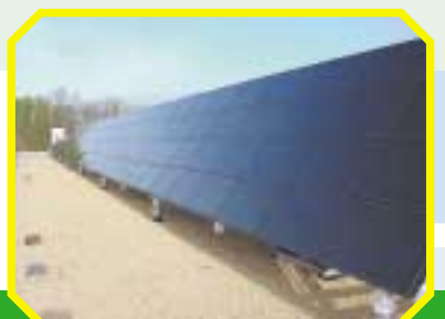
Part of a data logged Millennia array in Germantown, MD ▶
