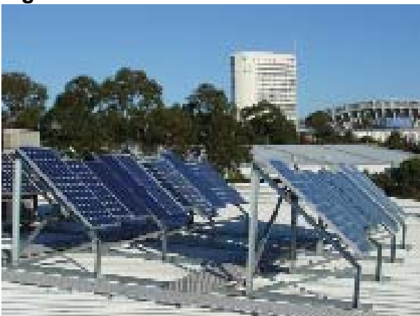
Fig 2 : Comparative module testing using IV sweep scanners in Sydney
