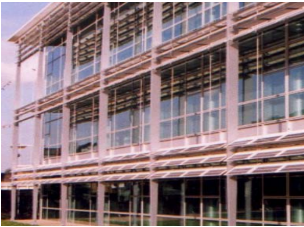
Fig 4 : BIPV Louvres in the UK
