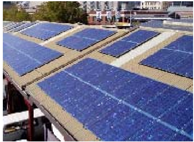
Fig 5 : Large Retrofit roof in Melbourne
